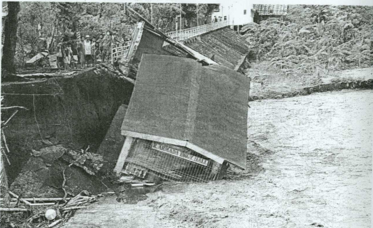
Residents looking at a damaged village hall after Typhoon Haiyan hit Janiway in central Philippines yesterday. Reuters pic
